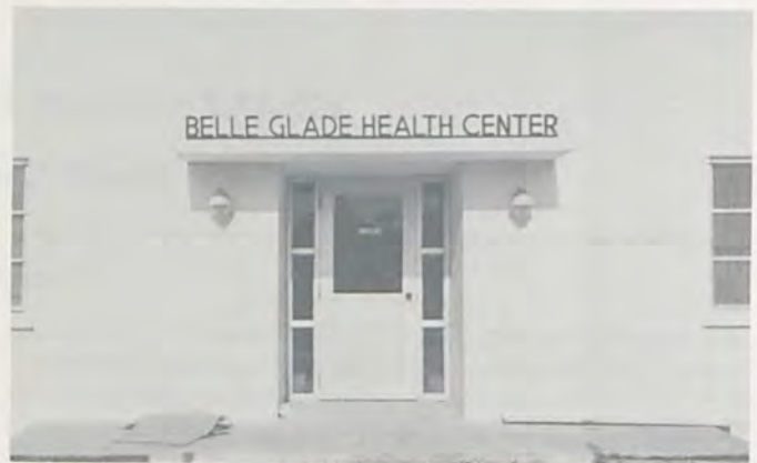
Entrance to Health Center.
